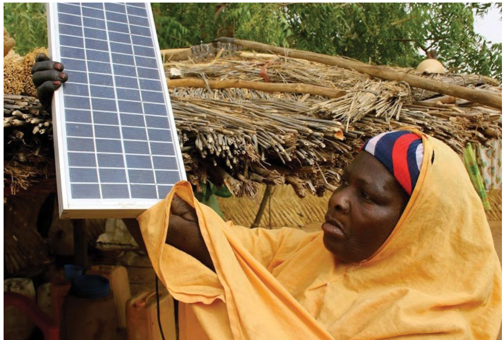
Installing a solar panel, Niger © Agnes Otzelberger / CARE
